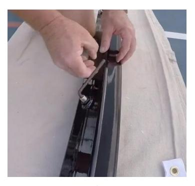
Step 5: Repeat step 4, by inserting one 1/2" stainless "Set Screw" into each of the end posts.
